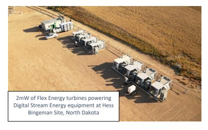
The Company has deployed an air-cooled portable data center at the Hess SC-Bingeman site southeast of Williston. These air-cooled units are at the mercy of North Dakota weather. The large swings in seasonal temperatures make server cooling difficult. Blowing snow causes problems when it enters the Portable Data Centers, and the high winds cause issues with cooling fans.
