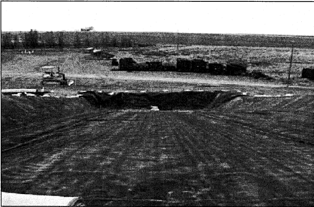
Figure 4: Geosynthetics in Lysimeter Pan
