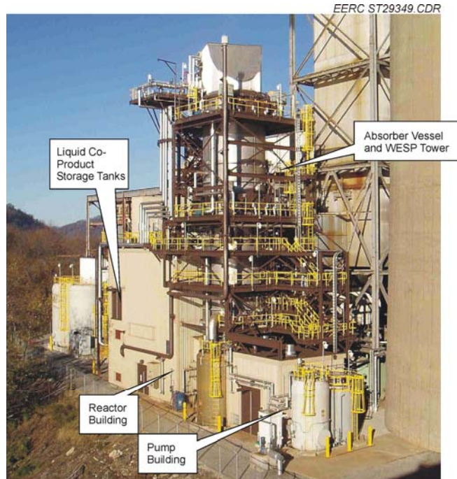
Figure 8. 50-MW ECO Burger Commercial Unit (BCU).
