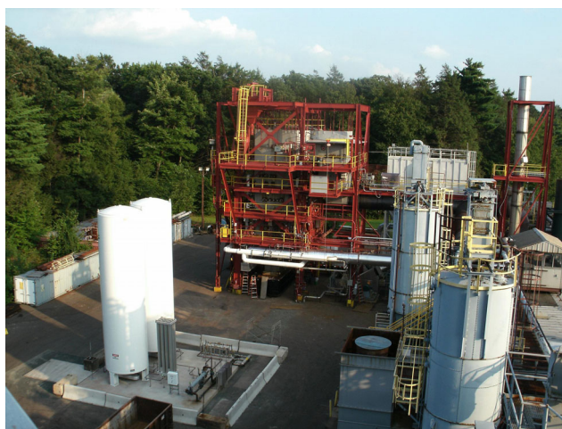
Figure 8 BSF with Modifications Installed
