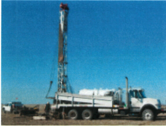
(A) Well drilling
