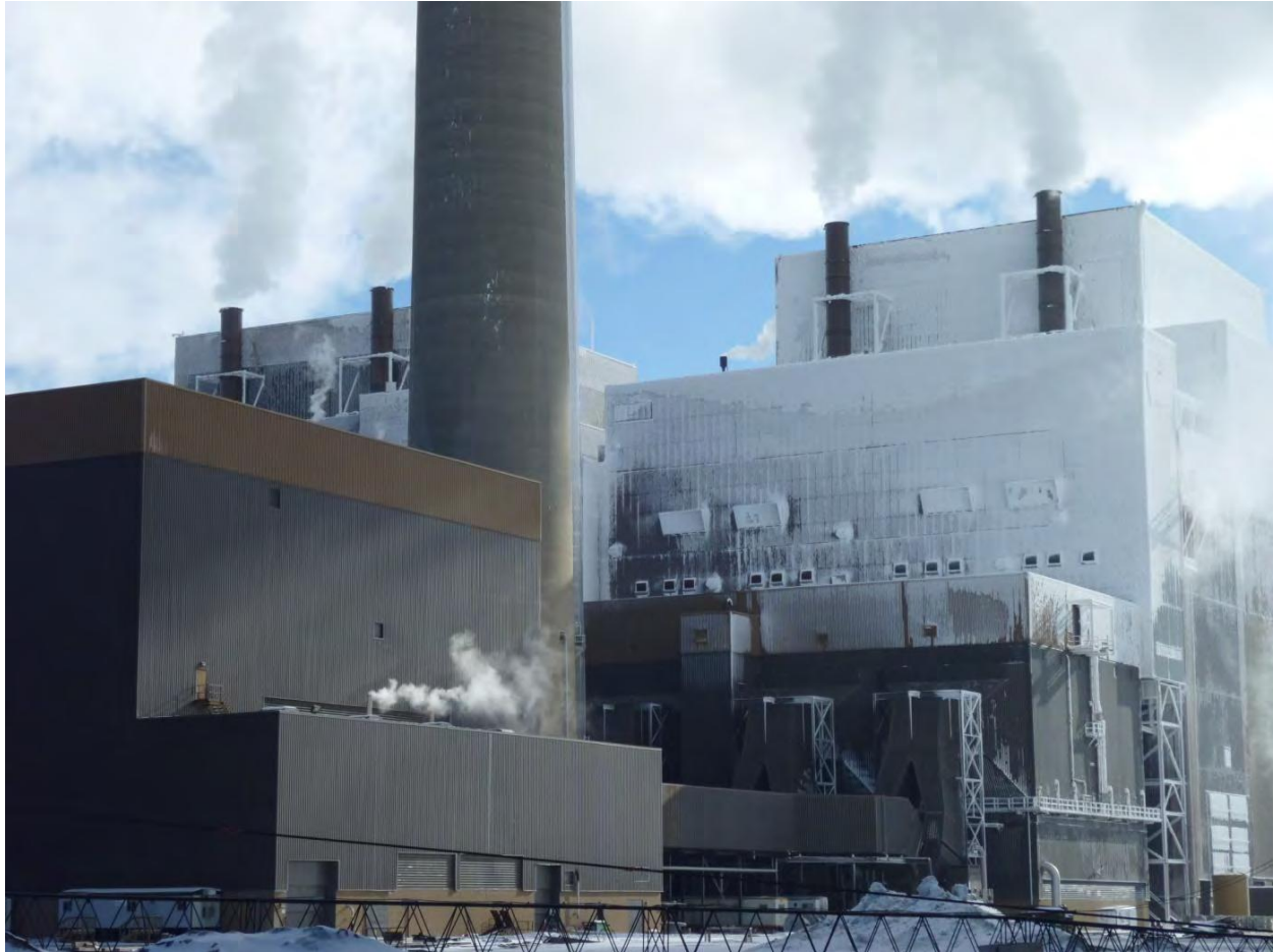
Figure 3-3 DryFining Dryers in Operation at Great River Energy Coal Creek Station
