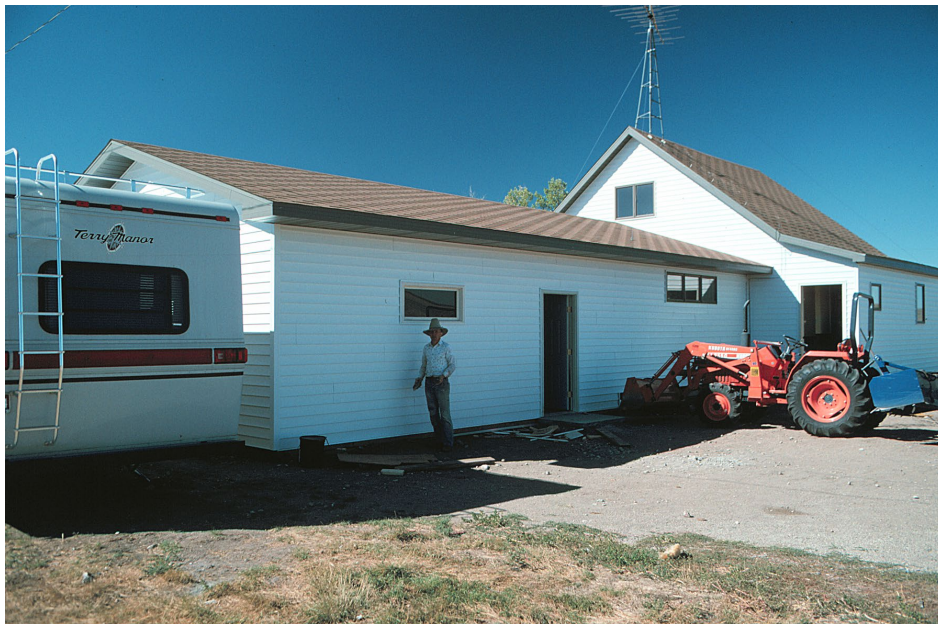
The local high school science teacher stands at the spot where woolly mammoth bones were encountered while digging the foundation. Photograph taken on August 25, 1988.
