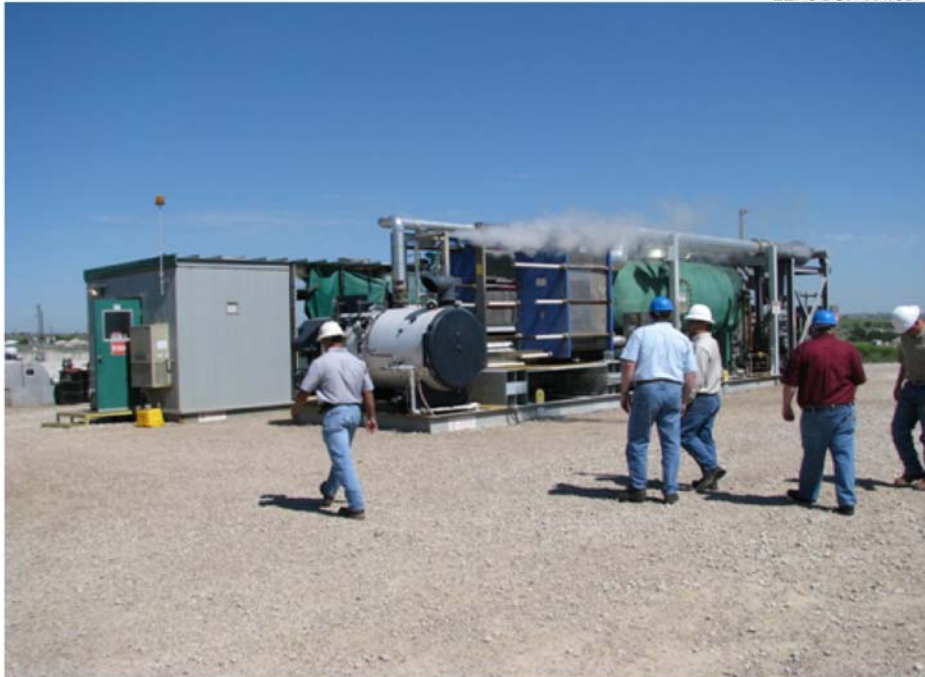
Figure 16. Aqua-Pure Nomad 2000 mechanical vapor recompression unit.
