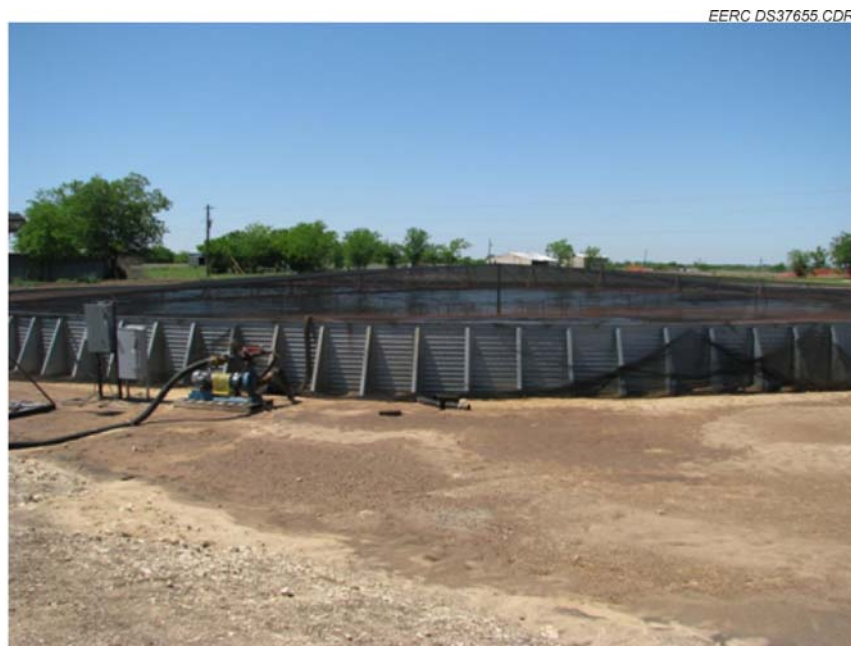
Figure 14. Frac flowback water storage impoundment.
