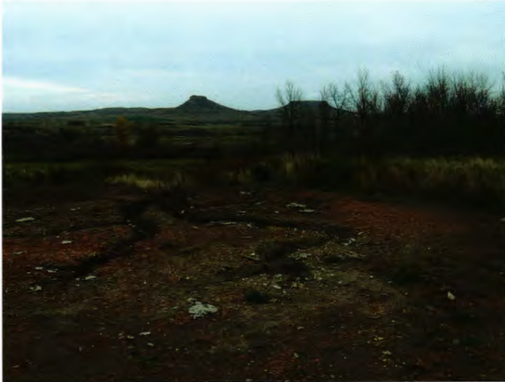
Figure 14: The H-408 is essentially without reclamation with the original scoria pad remaining.
