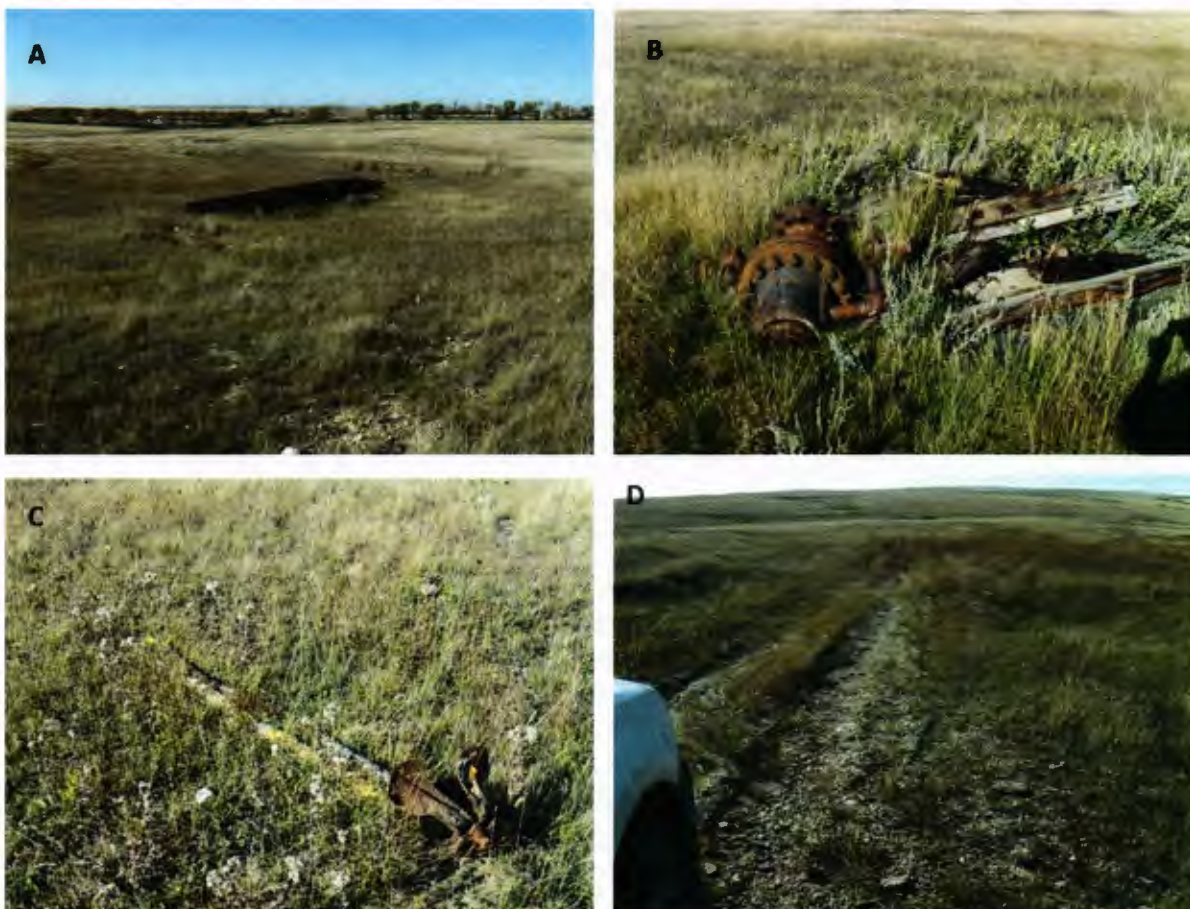
Figure 16: The N-152 showing residual infrastructure including the access road and debris piles. Vegetation was well established over most of the site and matched the ecology of the land adjacent to the former pad.
