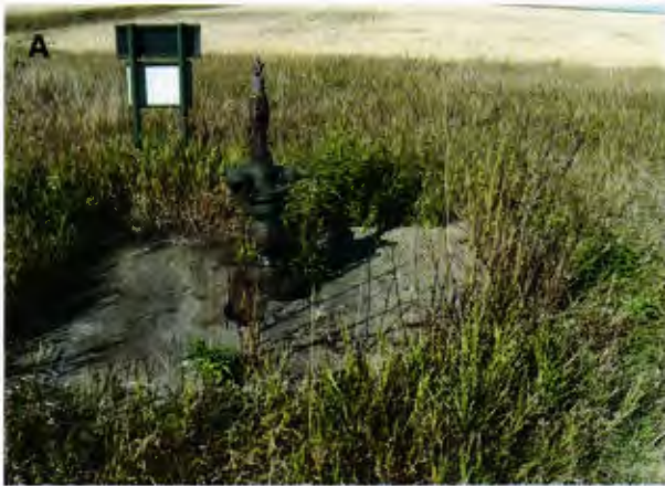
Figure 10: TMU F-144 residual infrastructure ranging from the wellhead to rig anchors. Overall the site was in good vegetative state and surrounding land was being used for production.
