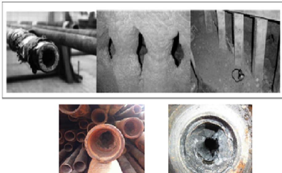
Figure B3: Scale deposition (left to right): in the pipeline, on a separator surface, on a clean separator surface, in downhole tubing, and in the riser pipe of a heating furnace. [6]
