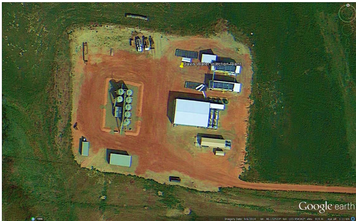
Figure 1.4. Davis water injection plant – ORC located in northeast corner of the site.
