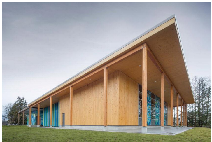
Figure 4: Example Community Pump House 14
