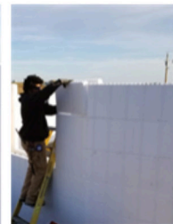
Easy to Stack ICF Walls
