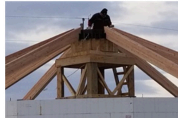
Installing Roof Beams
