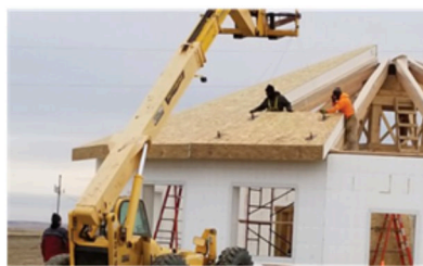
Adding SIPs Roof Panels
