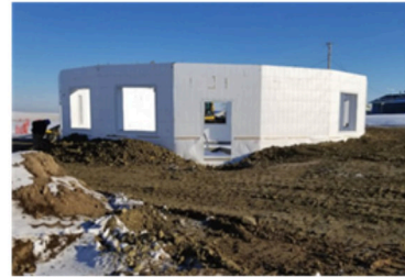
Completed ICF Walls
