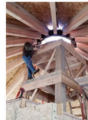
Removing Support
