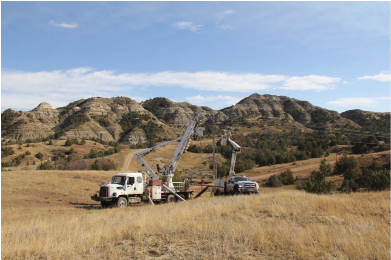
Photo courtesy Andrew Spratta – McKenzie Electric Cooperative
